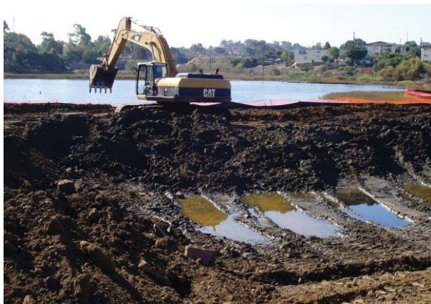
Digging the channel
