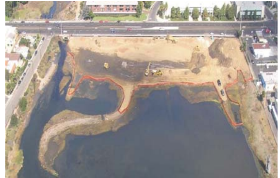
Overview of WPL Restoration Project, November 2005
